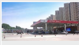
Qiuling Gas Station with optimizers (110 kW)
