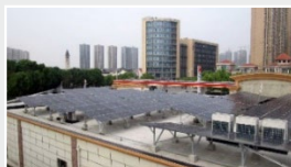
PetroChina Gas Station with optimizers (120 kW)
